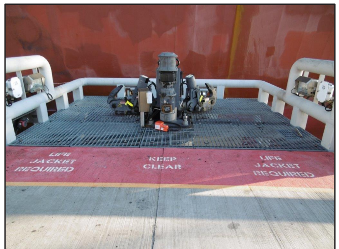
Figure 3: Mooring Hooks on Outer Wharf
