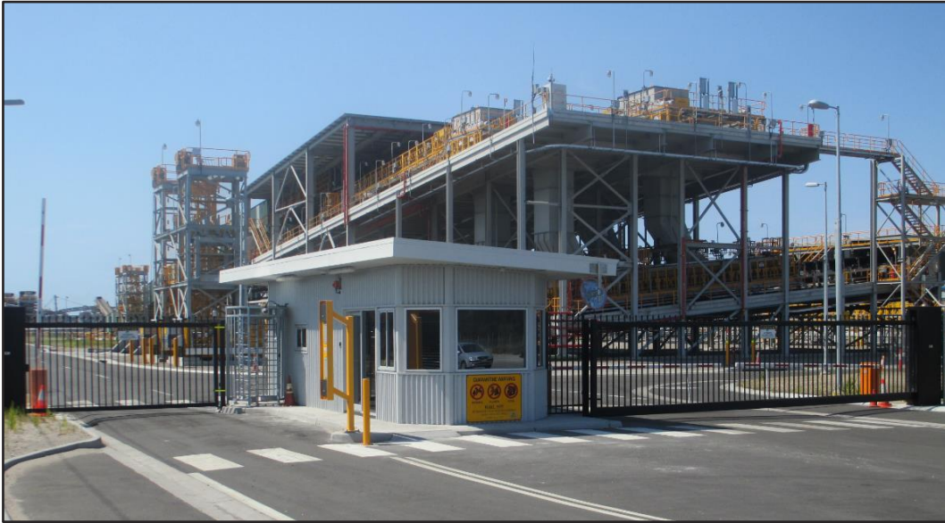
Figure 1: Entry to Wharf – Wharf Security Gatehouse
